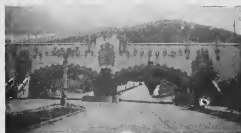
Lovers of stretches of good concrete road through beautiful country will appreciate this picture taken by Enrique Roze of the Plant Commissary when he was on a five week vacation in Venezuela to get married. The bridge is the Puente de Independencia and the road leads out of Caracas to Las Gachas, a newly finished housing development. Enrique also submitted a picture of a palm tree that was even crooked than the one printed in the last Esso News .
